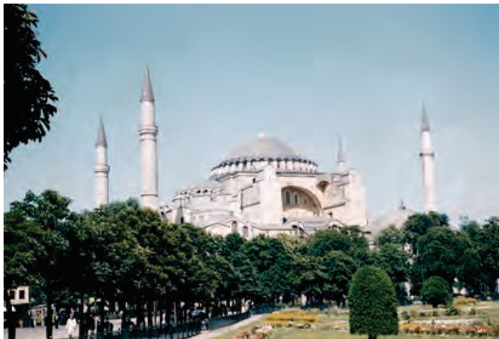
Figure 10. Hagia Sophia's four pencil minarets on the exterior. Anthemius of Tralles. 532-537 AD, Photographed: 1956. Hagia Sophia . https://library.artstor.org/asset/ABRMAWR_MELLINKIG_10310736414 .
