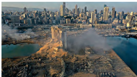
Figure 12. The aftermath of the Beirut explosion and the damage to the city 35
