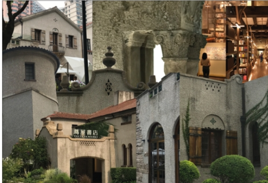
Figure 10. Collage by author of the Columbia Country Club after adaptive reuse. Note the distinct Spanish Mission Revival features that were restored during adaptive reuse, including the round arch windows, curvilinear gables, and stucco walls.
