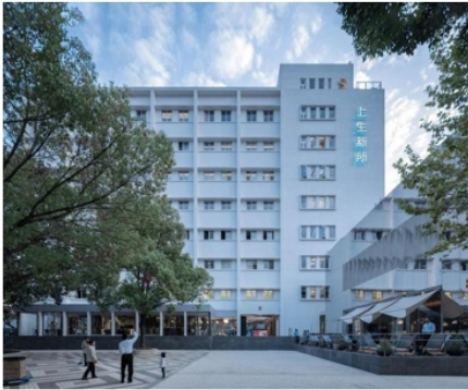
Figure 14. The refurbished MMR building looking out over the main square. To the right, the structure covered in mirror stainless steel is the former appliance building for the MMR building and has since been significantly altered to add dynamism to the main square (source: Thepaper.cn, 2021).
