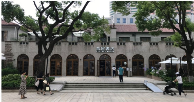
Figure 9. The Columbia Country Club's south façade after adaptive reuse; the south façade has been largely restored to its appearance upon completion in 1924, with the exception of the awning above the arcade. Photo by author.
