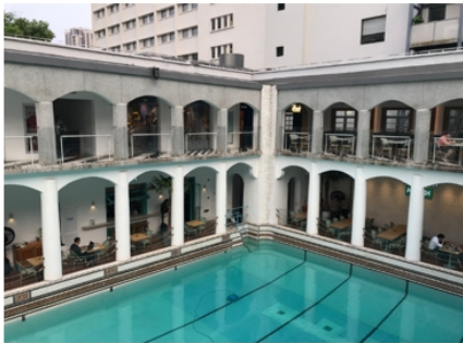
Figure 13. A corner of the Navy Club swimming pool. A stark color difference exists between the original colonnade and the colonnade added on the second level during the SIBP era. The colonnades have been transformed into an outdoor dining space. Photo by author.
